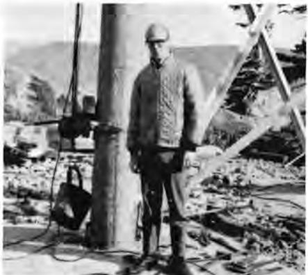
Above: Engineering's John Dixon, who engineered Claremont tower, visits site during construction to assist in the installation. Left: Lineman Wayne Benedict inspects reinforcing bars in one of three 10-foot holes dug out of solid rock before setting poles and pouring concrete for Claremont tower.
