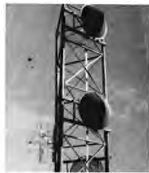
Left-right: One of the buildings near the Keddie depot can nearly be seen through legs of the reflector across the highway. The 30-foot tower on Sutter Buttes provides height enough for space diversity which assures that one of the antennas will always be receiving
