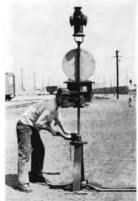
Switchman Mike Makuck throws switch to line track for engine and cut of cars being moved to another track to allow access by engine for coupling to assigned car.
