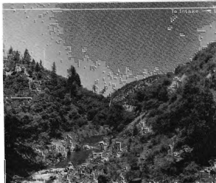
White line at top of picture indicates approximate location of double-decked railroad highway bridge across West Branch of Feather River. When back-filled, maximum water elevation will be about 900 feet. From railroad on lower deck to top of water line will then be 40 feet.
