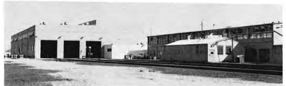
For running repairs and servicing, three tracks run through service bay above service pits
