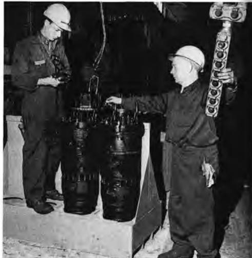
Machinist Helper S. G. Blake works on piston cylinder assembly as Machinist A. G. Rohde waits to lift unit by crane remote control.
