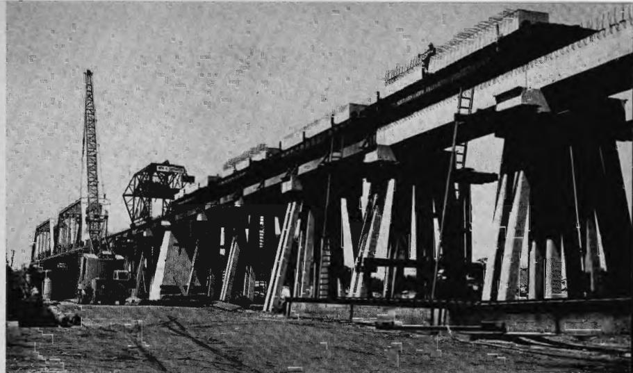
New bridge is higher and more strongly constructed to withstand future flood damage. Note pre-cast concrete girders atop flatcars ready for placement by gantry crane.
