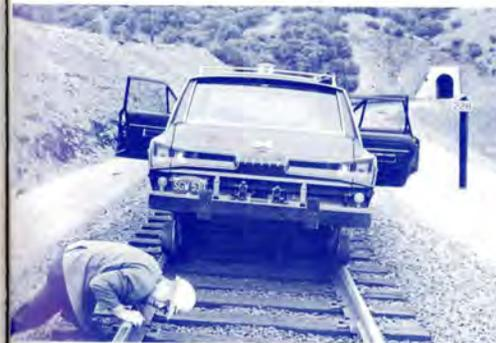
Milepost 228: Maury Crespo, engineer MW&S when picture was taken and now engineer administration, checks track alignment near 2,922.5 foot tunnel No. 5 shown in distance.
