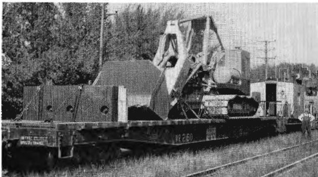
Over-all view shows redesigned flatcar with 96,000-pound KOEHRING SKOOPER and, on near end, a 21,000-pound counterweight used on rear of SKOOPER to balance weight of shovel when under load.
