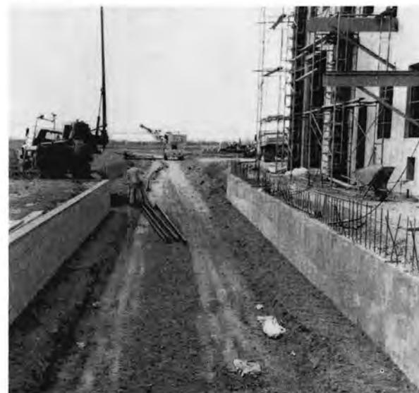
A depressed spur track leads from drill track to car-door-level ramp at Cook Paint building now under construction.
