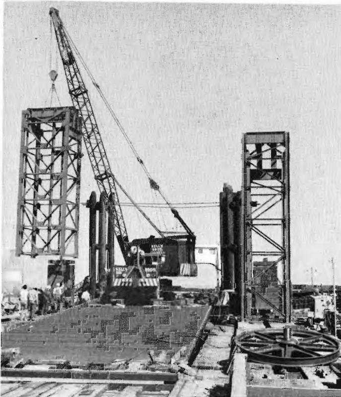
Left: Kelly Bros. crane with shortened boom drops gallow frame over counter weights. Bull wheel, right foreground, is one of two used to support main cable for lifting apron.
