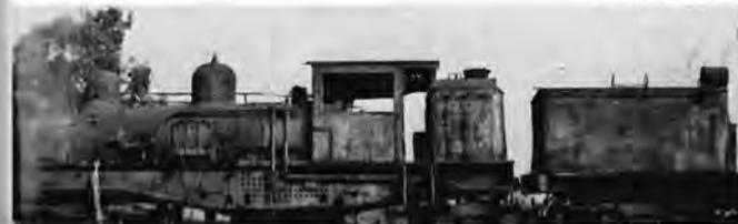
Left: With a unique gearing system this 65-ton Shay, built in Ohio in 1920, once pulled Yosemite Lumber Co. logging trains up grades as steep as 14 per cent.
