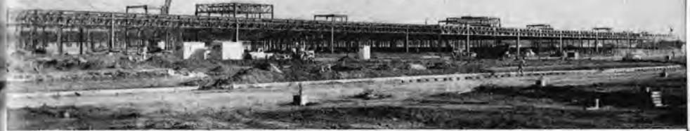
Engineering "news" was made last month when Western Pacific's main track on the San Jose branch was cut, three large diameter culverts installed, and the line restored to service, all in an elapsed time of 14 hours.
