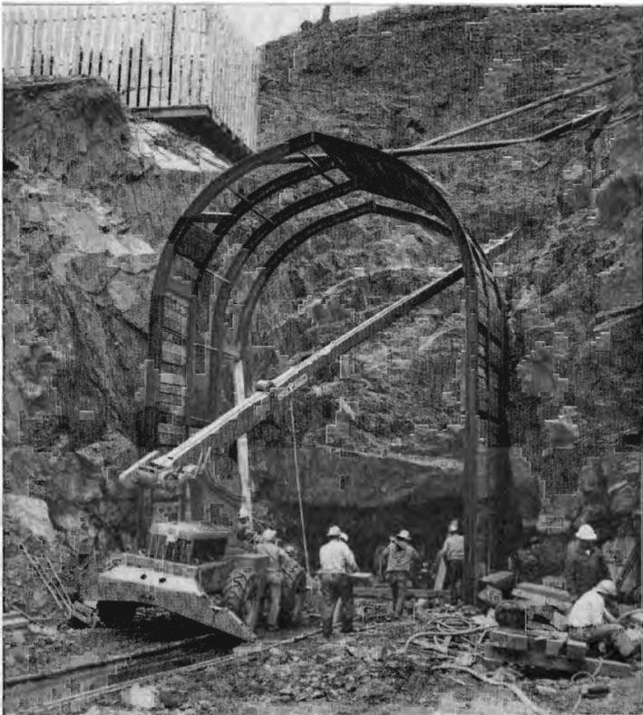
Relocation of WP's main line around proposed Oroville dam is in full progress. This Department of Water Resources photo shows one crew installing tunnel ribs for temporary support at the west portal of the 8,800-foot-long Tunnel 5 in Dark Canyon. Construction work is being done by Peter Kiewit Sons' Company.
