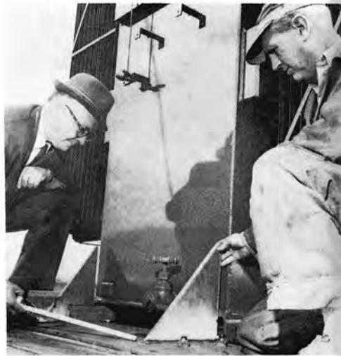
They then checked and found that gusset plates were uniformly placed to best support and anchor the transformer to car deck.
