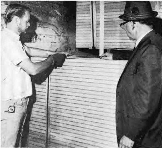
Cliff suggested Operator Bob Pittman insert plywood under strap to prevent cutting hollow core doors at Stockton Door Co. plant.
