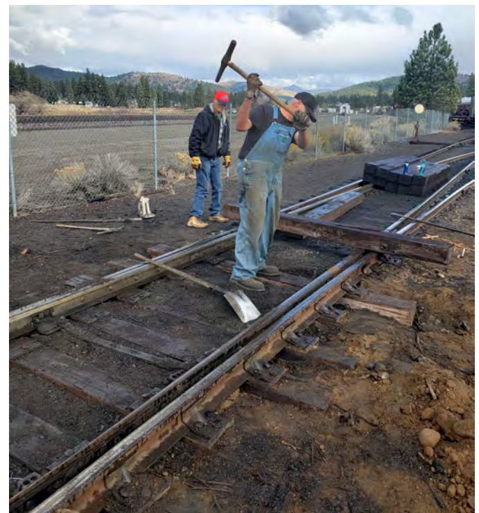
Above: Roger Stabler spiking ties in the Rip Switch - Photo by Greg Elems 11/16/23
