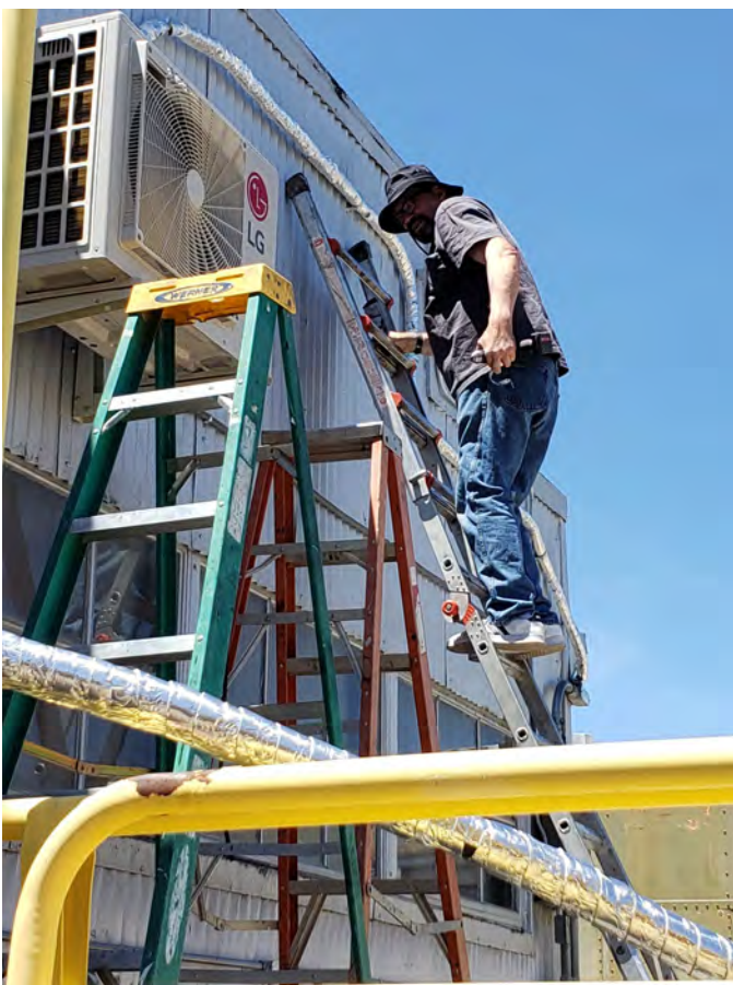
Eric McKay, Don Nelson and Eugene Vicknair teamed up on finishing the new A/C - heater units for the Museum Store. Eric is seen here working on it.
