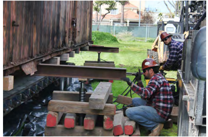
Lifting the 55069 off the trailer.
