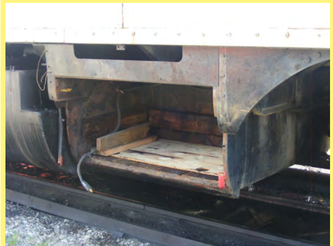
WP 917's right side battery box, prior to cleaning. Regular cleaning helps slow the corrosive effects of battery chemicals on the metal of the locomotive. The wood lining prevents terminals from inadvertently touching the metal body.
