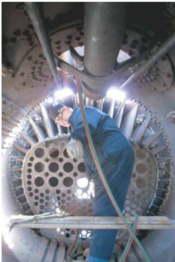
Roger Colton removes rivets from the rear tube sheet.
