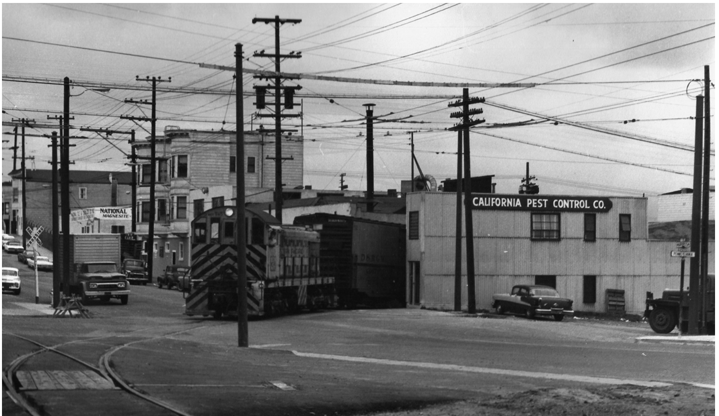
FROM THE PAST - A WP Alco S2 pulls a cut of cars across Mariposa Street in San Francisco. The train is leaving joint Southern Pacific - Santa Fe rails and about to roll onto Santa Fe tracks. This is all part of the trackage rights WP obtained in 1962 to bypass burned out Tunnel A. - FRRS Archives
