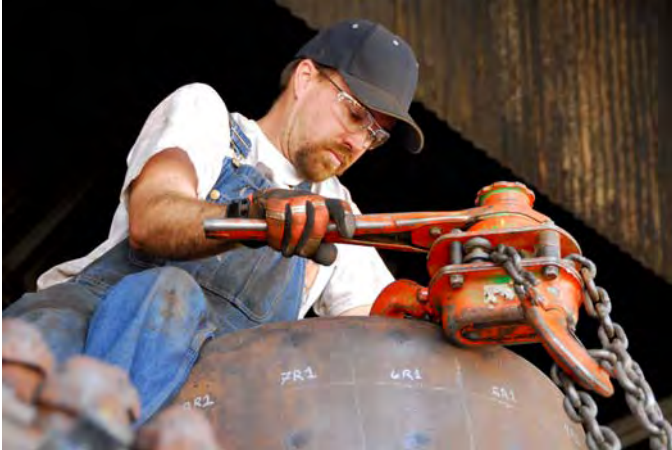
Erin Swain checks the rigging for lowering the power reverse from the side of the boiler.
