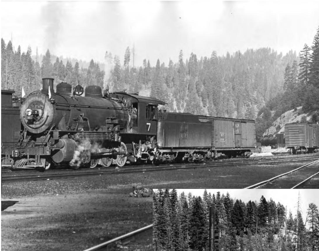
WP 7, a 2-8-0 built by Baldwin in 1906, switches a train in the Feather River Canyon, specifically at the east end of Keddie. The roundhouse, shown in the photo below, is right behind the photographer. This class of engine was the first received new by WP.
