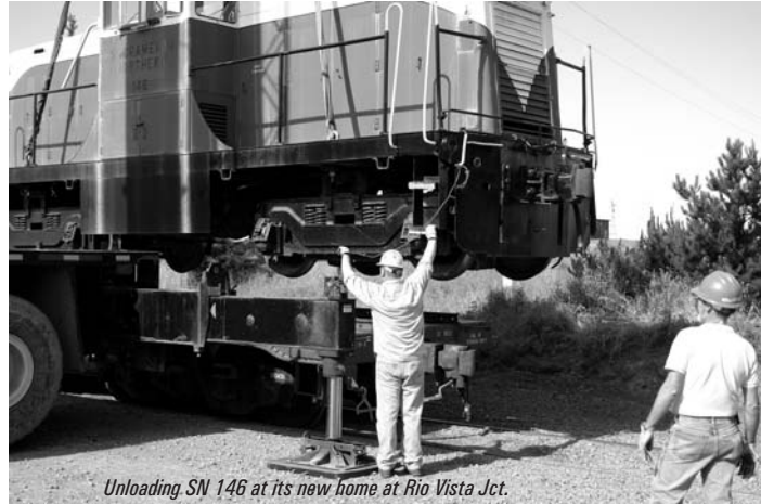
Unloading SN 146 at its new home at Rio Vista Jct.
