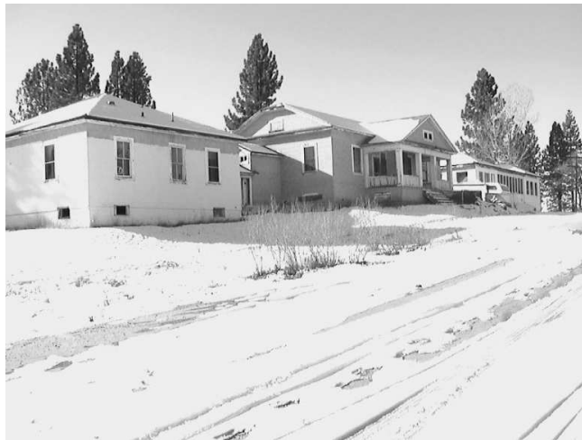
A cold December morning shows the hospital as it looks today. With work, grants, and effort it will be rebuilt. -Jim Murphy photo
