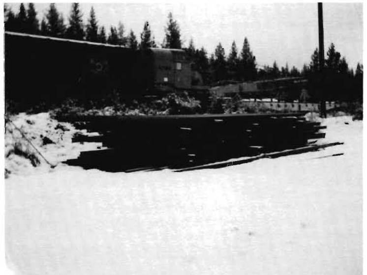
Two truck loads of rail from Grays Flat, consisting of 108 pieces of rail, and weighing 55 tons, are stacked inside the balloon track for use on possible track extensions at the Museum. Some rail dates from 1907 when WP was built. Photo by Norm Holmes.
