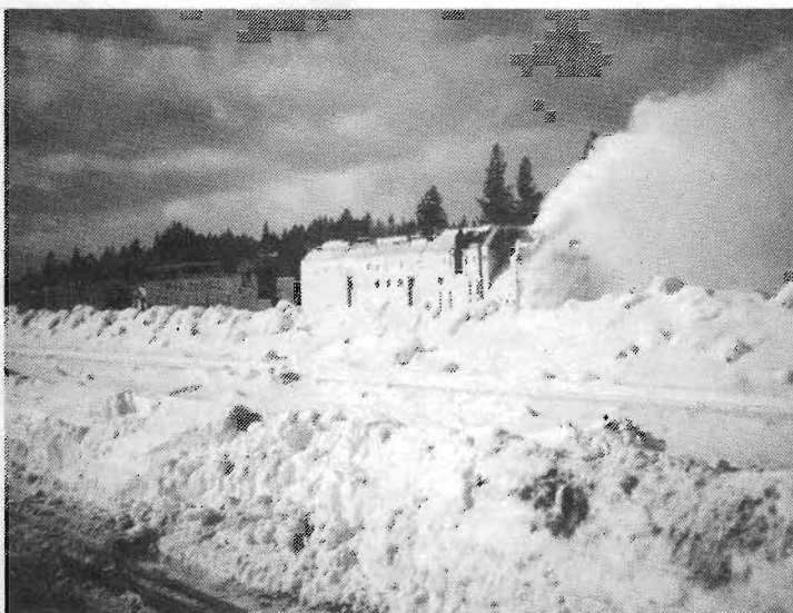
Union Pacific sent one of their three remaining rotaries from Cheyenne to Portola. It is shown here clearing the UP Portola yard, which is the first time a rotary has been used in Portola since the winter of 1970-71.
