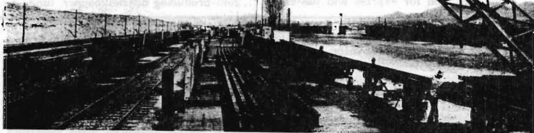
General view of loading area. At left, carloads of 39-foot rails just arrived from mill. In foreground, 78-foot rails are loaded onto cars destined for track-laying installations.
