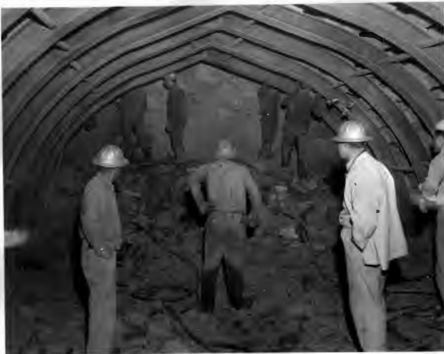
No. 188-5 10-25-58 Tunnel No. 4 (W.P.R.R. No. 7). Placing final lagging prior to holing out of Portal 4W.
