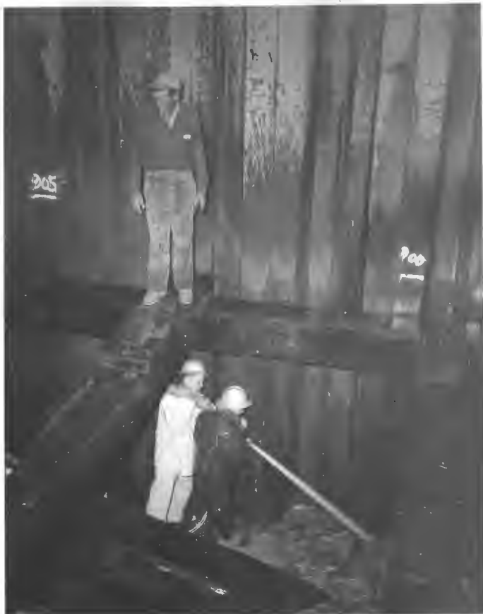
No. 191-1 10-16-58 North Fork Bridge. Washing down bedrock before placing reinforcing steel at Pier No. 3.
