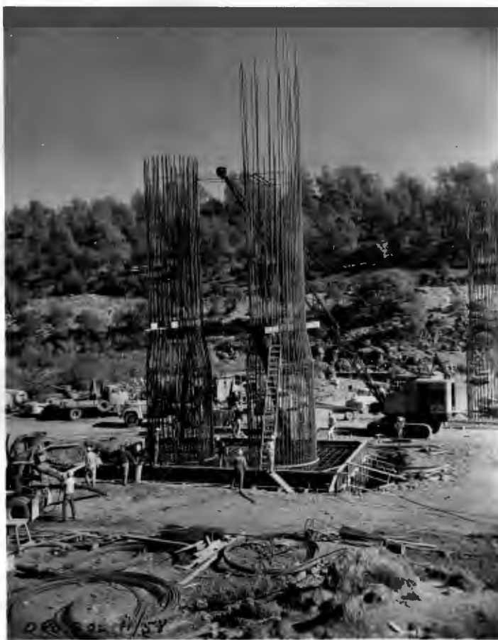
No. 202 11-7-58 Feather River Bridge. View showing men and equipment at work placing concrete on Pier No. 8.
