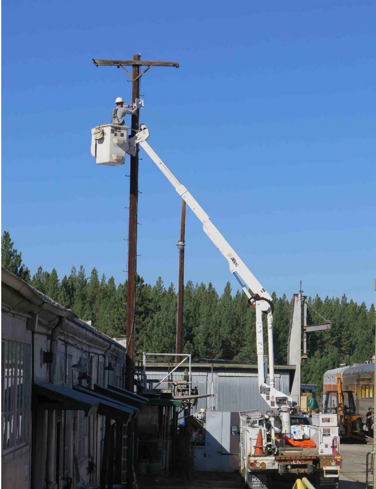
PST Employee Austin installing the antenna for the new system
