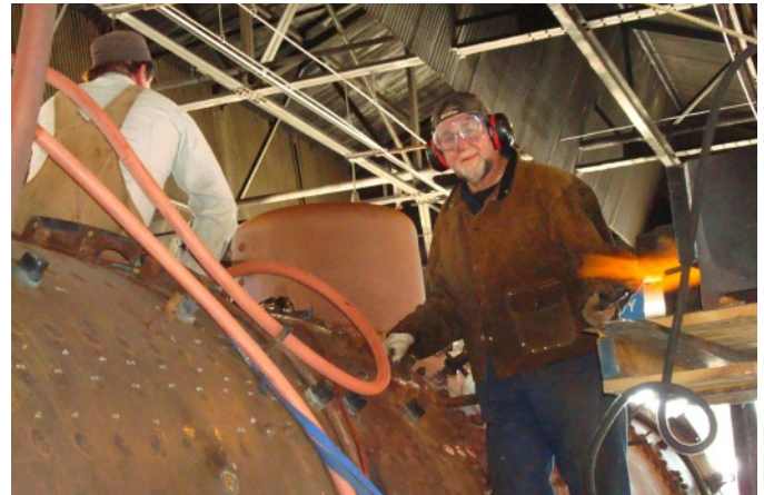
Kirk Baer prepares to pass a hot rivet.
