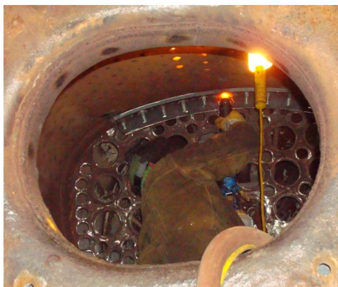
Norman riveting into the knuckle patch.
