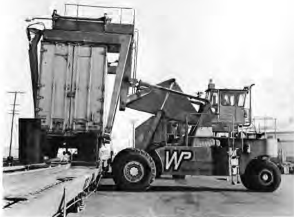
The "piggy-packer" with arms extended can unload vans (or trailers) with the same ease it can hoist a container from or to the railroad flat cars. These cars are designed to handle both vans and containers for the railroad.
