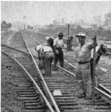
Seldom in the news, but important to the successful operation of Western Pacific trains, are WP's section gangs. Manuel Olivera, foreman, and Section Gang 3, replace ballast at Mile Post 30, just east of Niles station. Manuel has been with the company nearly 30 years, 24 as section foreman at Niles. Other members of the gang are: E. Ramos, A. Cocoa, P. Vega, J. Lara, and J. Ojeda.
