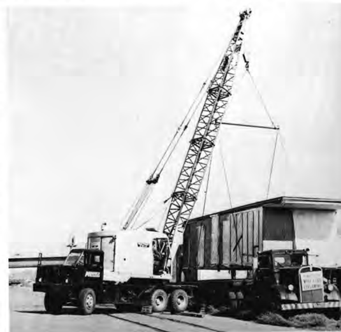
A roof section is joined to the walls of this Boise Cascade housing module at Meridian.
