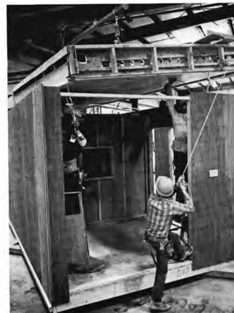
A roof section is joined to the walls of this Boise Cascade housing module at Meridian.
