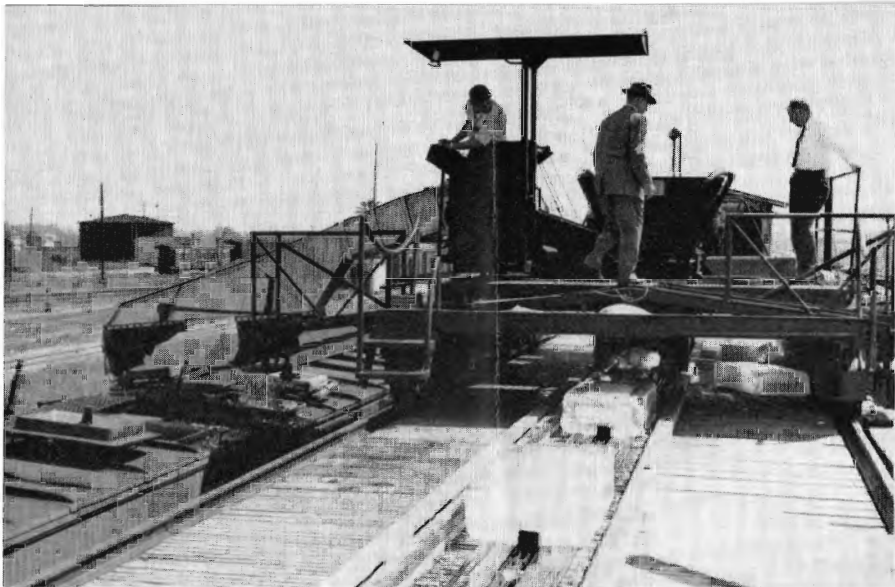
Taken from icehouse side of ice-machine, picture shows blocks of ice riding conveyor line
