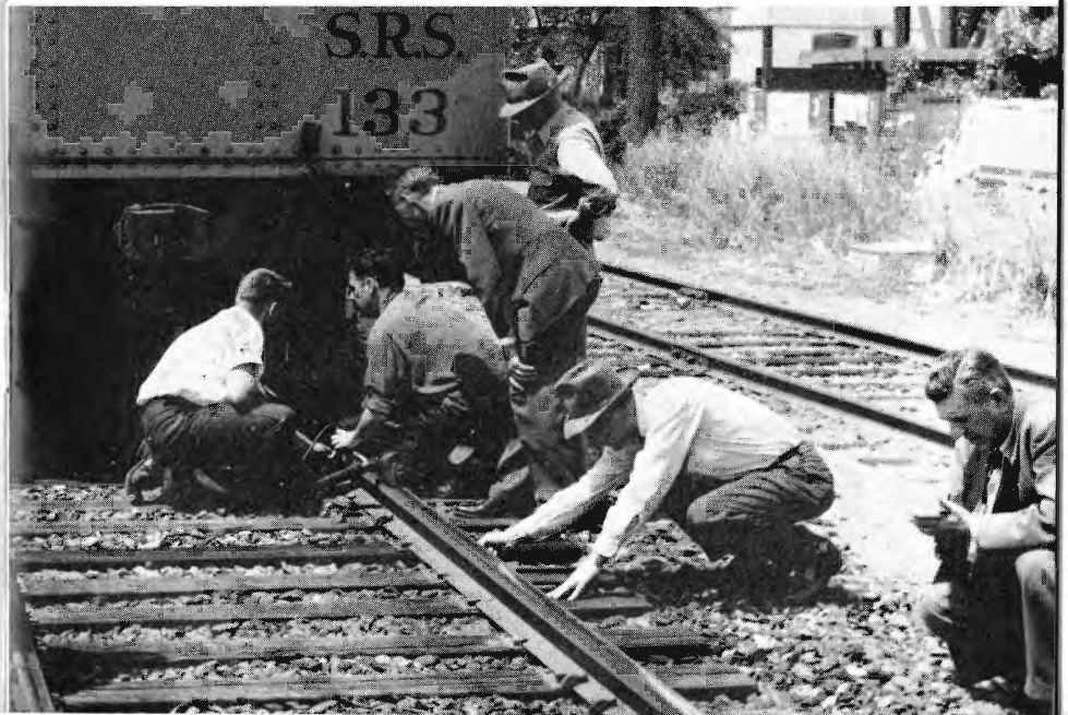
Crew members and WP engineers make further test of rail recorded defective by instruments aboard the car. Trainmaster R. A. Henderson leans over to read heat number stamped on rail by manufacturer to Roadmaster John Connelly, taking notes (far right).
