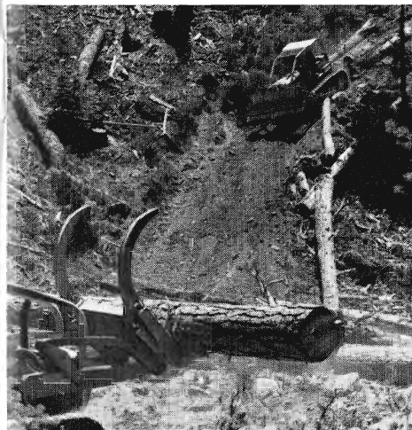
Below: "Turn" of logs comes down skid trail to log landing, as cat grapple in left foreground scoops up log to be piled near log truck station.
