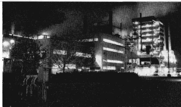
Fibreboard's San Joaquin Pulp & Board Mill at night. A newly added recovery boiler is at the right. Power house is in the center.
