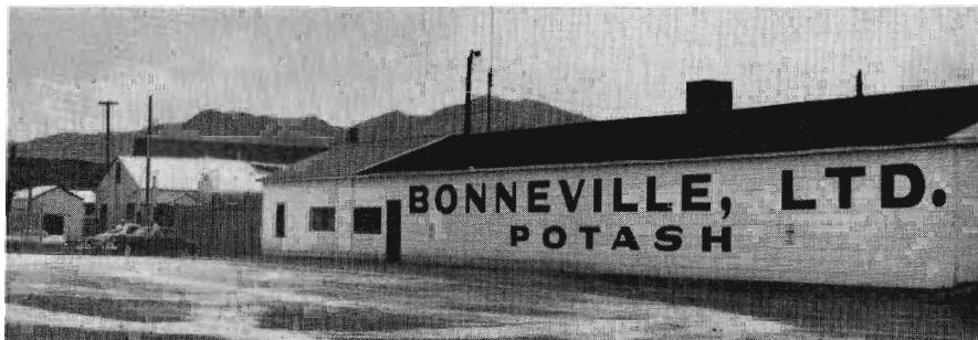
Bonneville's office and spare parts warehouse at Wendover, Utah. Flotation mill is in rear.
