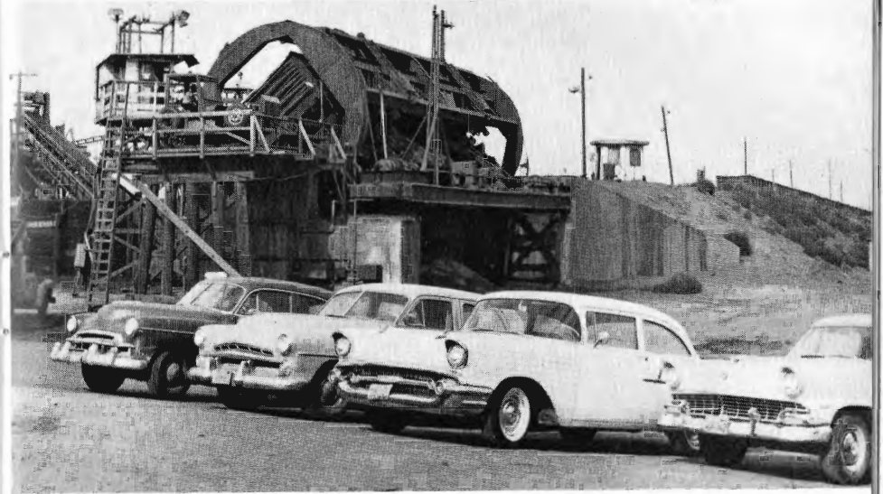
At Port of Stockton loaded cars at upper right wait their turn to be emptied by means of a revolving car dumper. In upper left background potash moves to ship on rubber-belted escalator.
