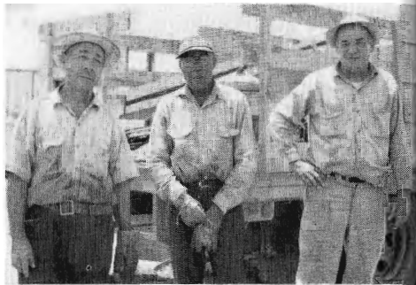
Manuel Ramirez, Garther Price, and Extra Gang #2 Foreman August J. Ackerman, on lunch break while installing siding for new W. P. Fuller Company glass warehouse at Decoto, California.
