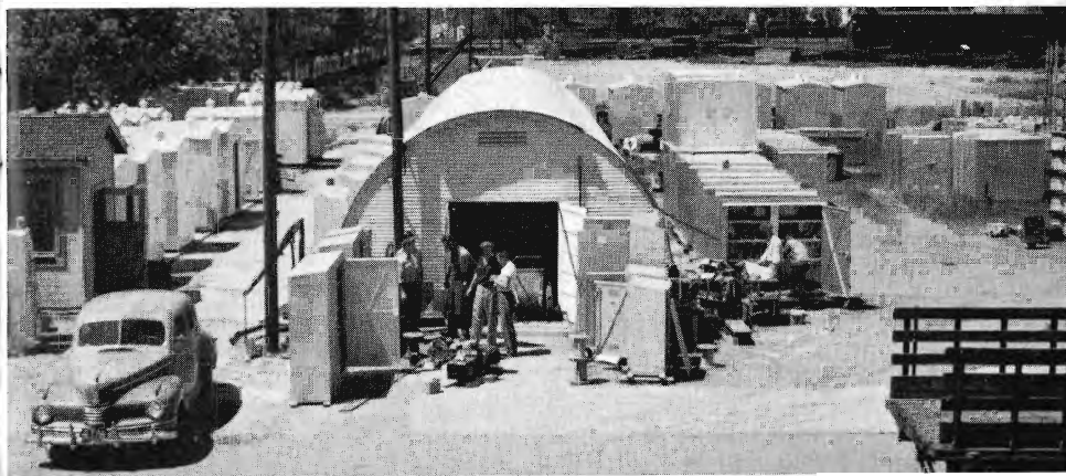
General view of the signal department shop facilities at Sacramento.
