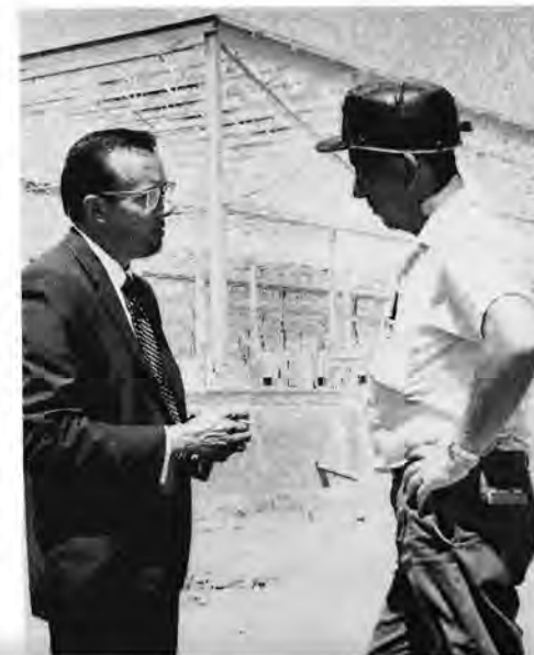
Dick Hocker, assistant to director of industrial development (left) checks the Reynolds' plant progress with construction engineer.
