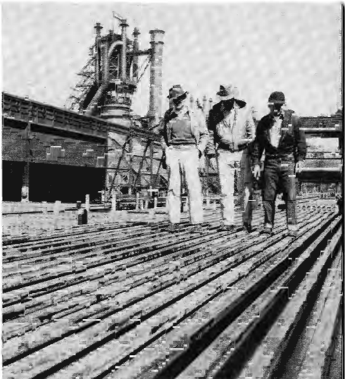
Walking on top of a rail is against all railroad safety rules, as WP railroaders know. But these "rail walkers" find it relatively safe, as the rail surfaces have not yet been polished by train wheels. These rails are being inspected, first on the upturned bases, then on the heads, by Ed Batchelder, WP, and George Boedecker and Al Niznich, of CF&I.
