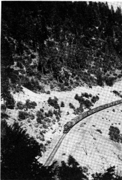
Photograph by Frank W. Taylor, retired WP engineer (Eastern Division 1910-42), from Feather River Highway near Keddie, vintage 1939.
