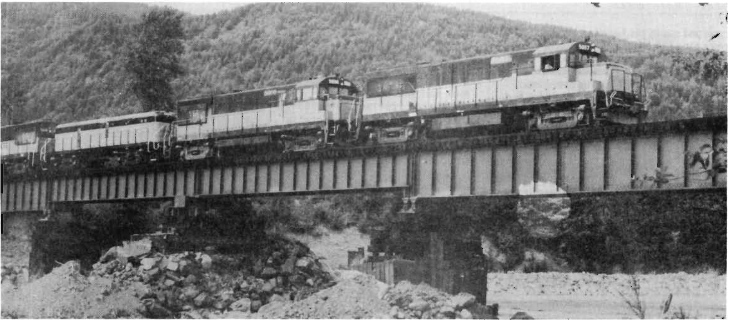
5057 leads Eastbound Morton Logger across Nisqually River Bridge Aug 6, 1978
