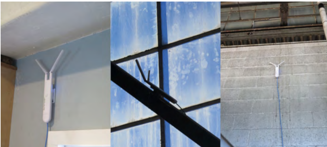
New Museum WiFi installed by Kenneth Finnegan & Kerry Cochran. Access points are now in the Silver Debris (crew lounge), southwest corner of diesel shop and near the Museum Store - photos by Kerry Cochran
