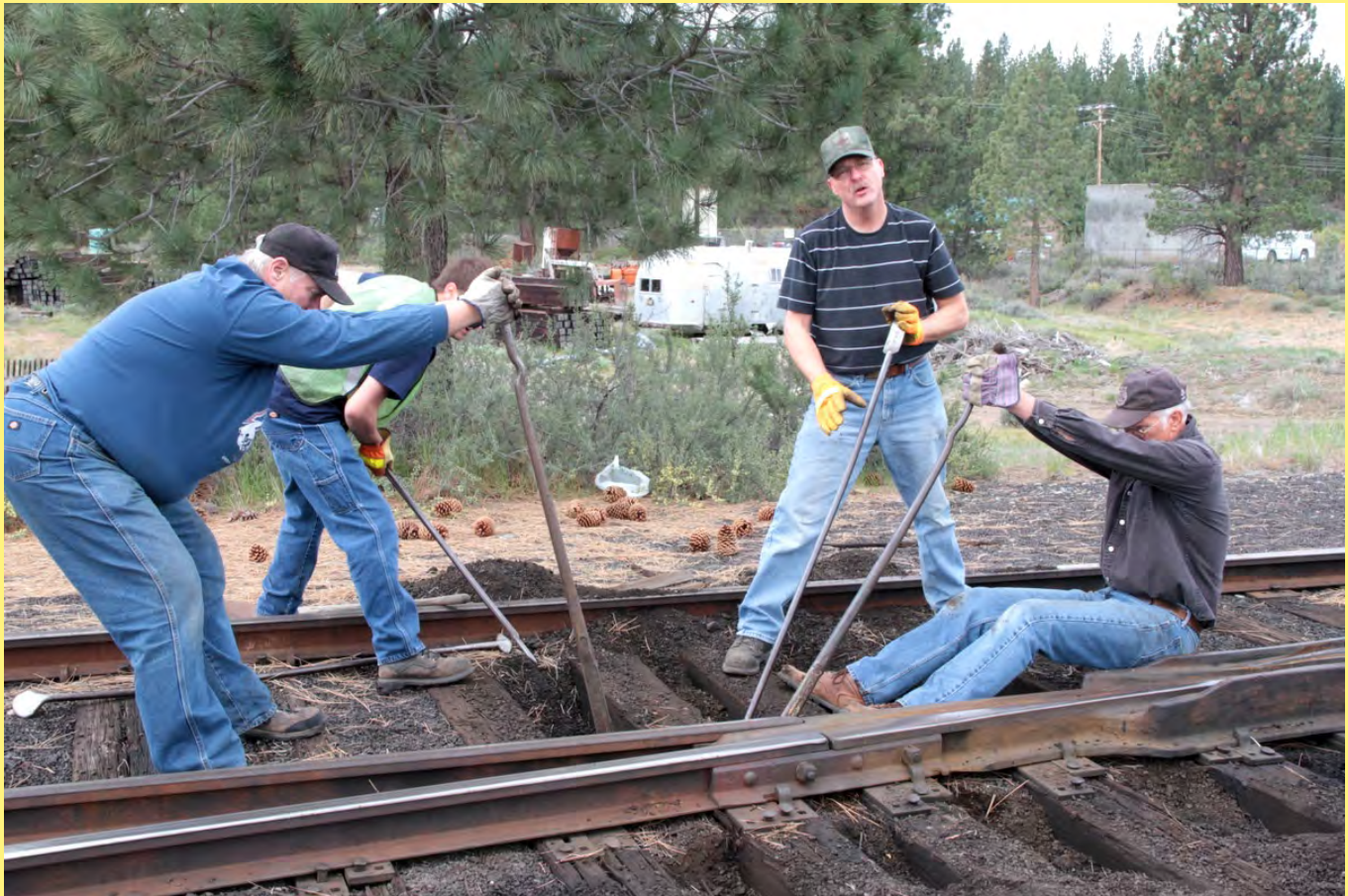
Greg Elems explains the efforts of volunteers doing track work to the photographer on 10 May, 2014. The ties under the switch frog are being raised and tamped to correct settling that has occurred over time. Pictured left to right: Rick Gruninger, Matt Elems, Greg Elems, Duane Vander Veen.
