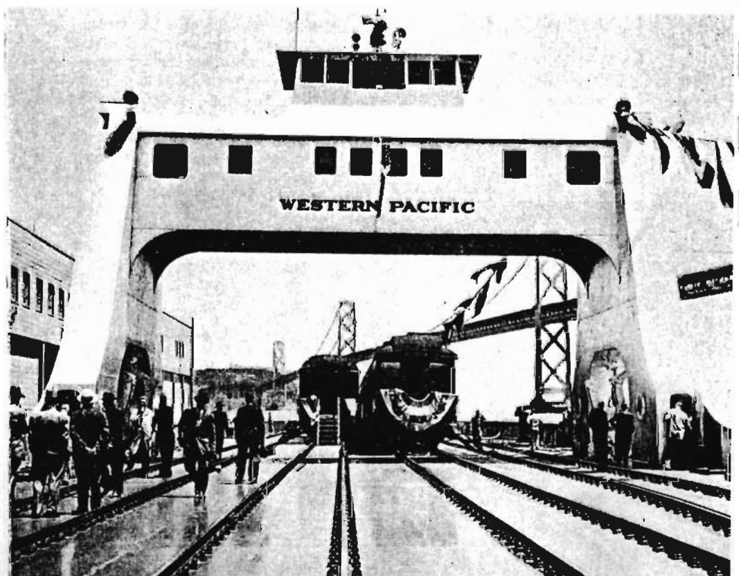
From her deck the vessel's single-span bridge amidship makes an impressive sight. She can handle 28 freight cars on her 375-foot deck.
