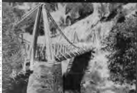
Suspension Bridge at Bidwell
