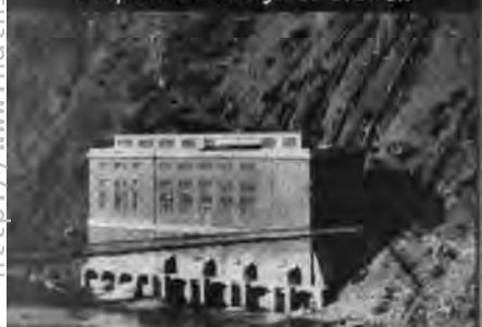
P. G. & E. Power Plant at Las Plumas
